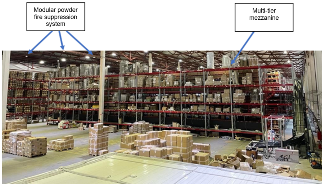
Fig. 2. Warehouse with multi-tier mezzanine
