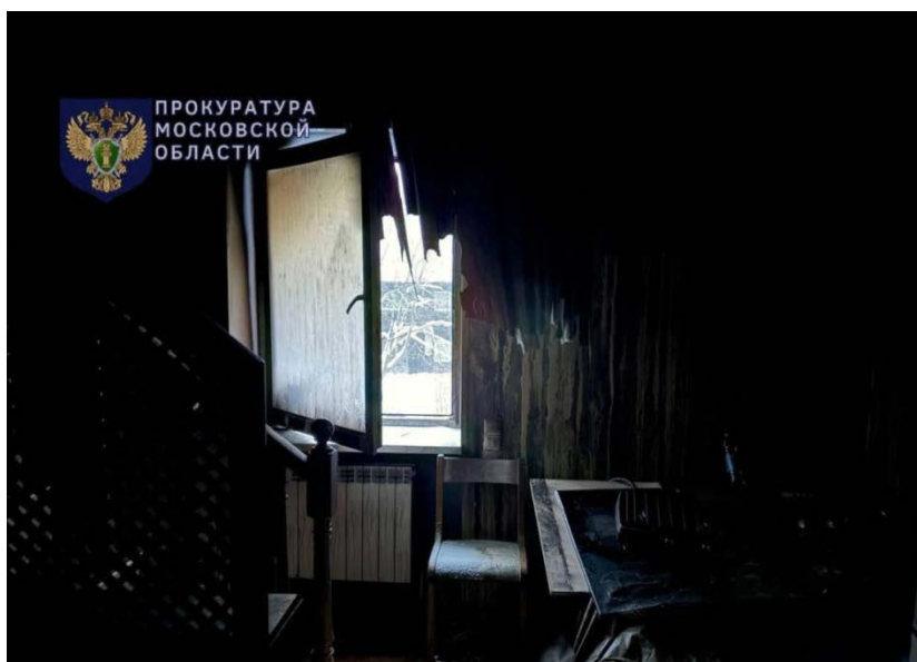
Fig. 5. On January 27, 2026, a fire broke out in an illegal hostel located in a private residential building in the Moscow region, killing four people
