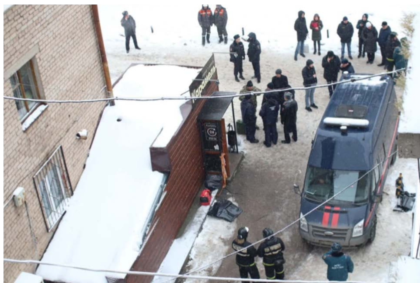
Fig. 2. On January 20, 2020, the heating pipe of the Caramel mini-hotel burst in the basement of a five-story residential building in Perm
