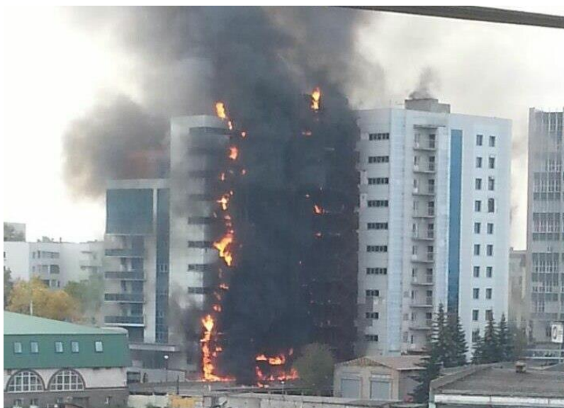
Fig. 2. Fire in the building of the business center of the Bashkir generating company
